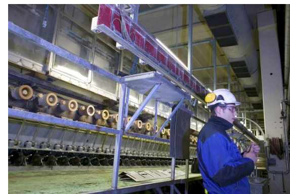
Access to full-scale plant
